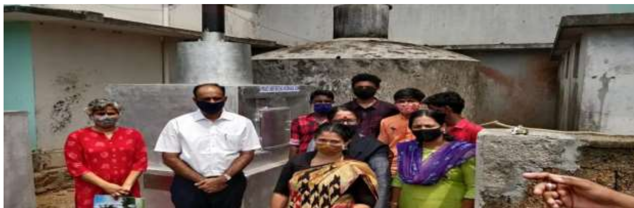
Waste Burning Incinerator installed and commissioned at school premises
